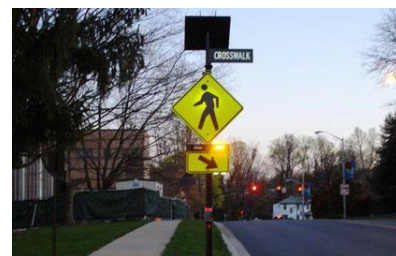
Rectangular Rapid Flashing Beacon
