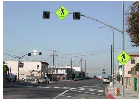
Overhead Flashing Beacon
