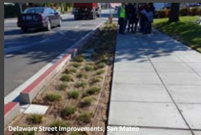
Delaware Street Improvements, San Mateo Source: CDRA, 2014
