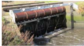
Bayfront Canal/Flood Slough Weir (Moffat and Nichol, 2012)
