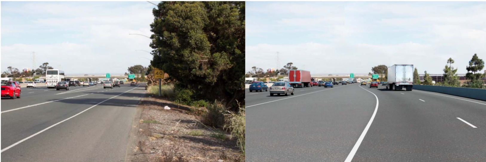
Example of ramp realignment at southbound off-ramp at Holly Street, San Carlos
