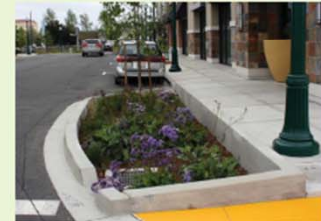
▲ Stormwater curb extension frames corner bulbout.
