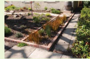
▲ EXAMPLE: An example residential stormwater planter that captures roof runoff first into a rain barrel and an excess runoff is directed to a stormwater planter.
