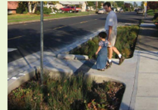
▲ Example mid-block stormwater curb extension.
