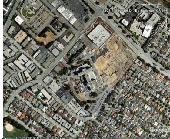
Mills-Peninsula Hospital, showing excavated area for new construction.
