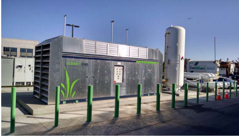
Figure 24. SSF Scavenger Company CNG Fueling Infrastructure
