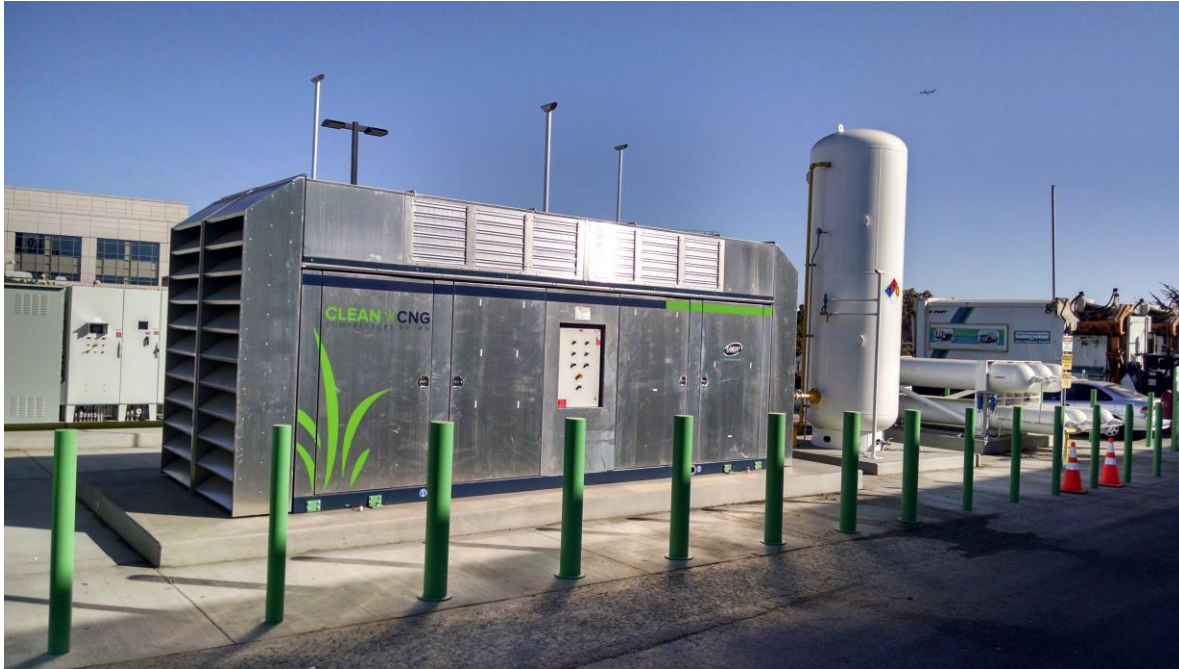
Figure 7. SSF Scavenger Company CNG Fueling Infrastructure
