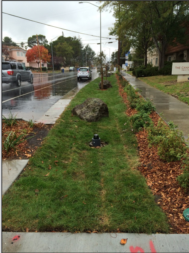
Hacienda Avenue: Failing pavement, unsafe large ROW
