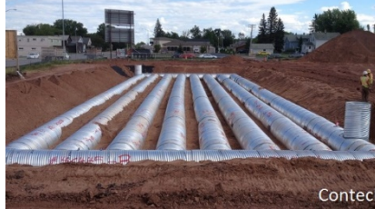
Example corrugated metal pipe configuration
