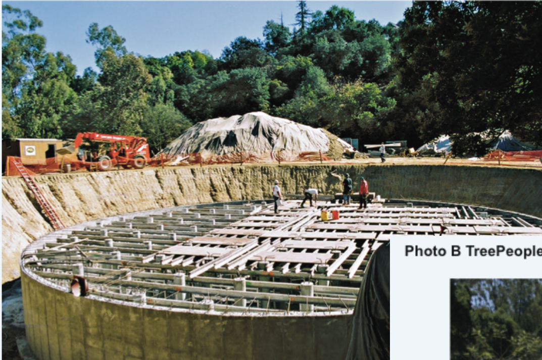
Photo A TreePeople's 216,000-Gallon Cistern Under Construction
