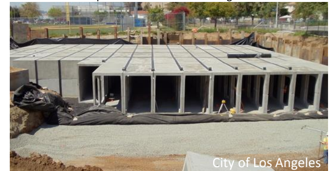
Example concrete chamber configuration
