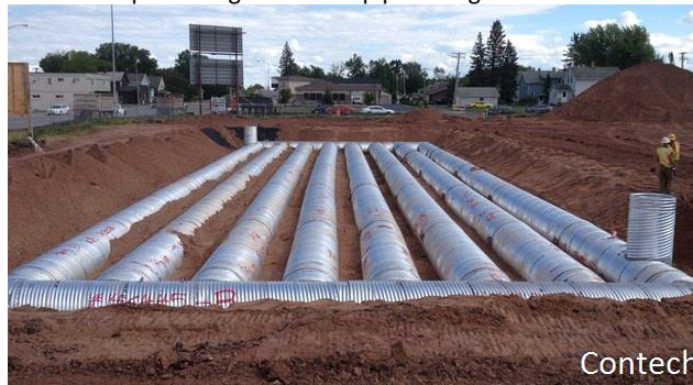
Example corrugated metal pipe configuration
