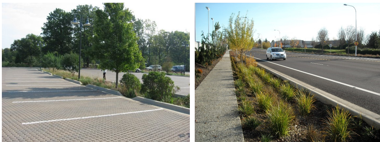
Figure 4-3. Example permeable pavers with bioretention cell at a parking lot (SMCWPPP 2009) and a vegetated swale along an arterial street (SMCWPPP 2009).
