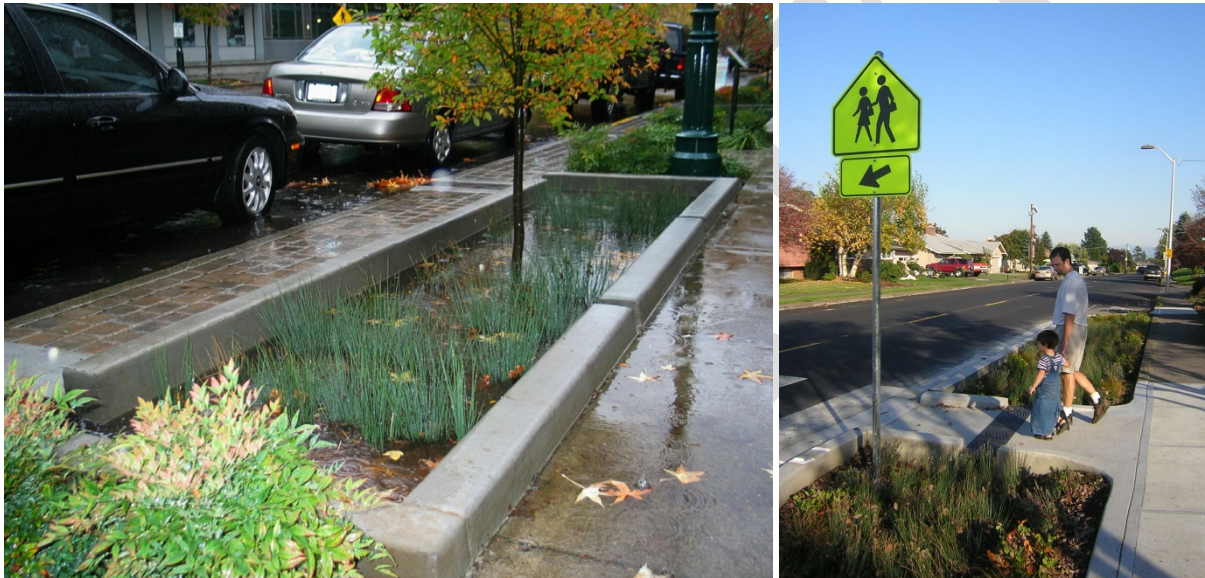
Figure 4-2. Example stormwater planter box (SMCWPPP 2009) and bioretention curb extension at a crosswalk (SMCWPPP 2009).
