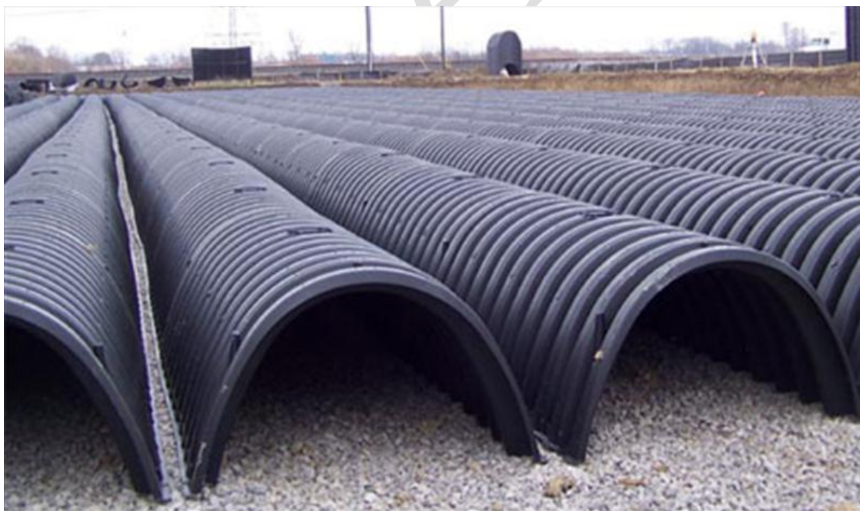
Figure 4-1. Subsurface infiltration system installation under a parking lot (SMCWPPP 2014a).
