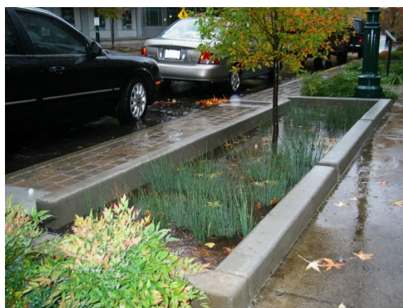
Figure ES-2. Example green street with stormwater planter box (SMCWPPP 2009)
