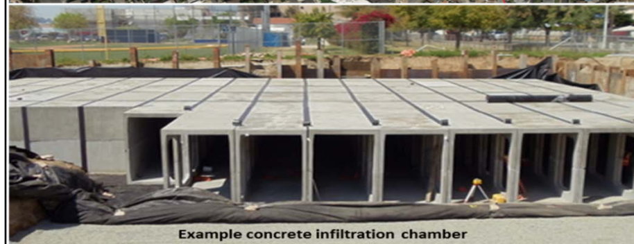
Example concrete infiltration chamber
