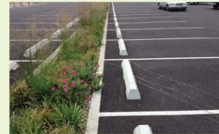
▲ A stormwater planter within the interior median of a parking lot.
