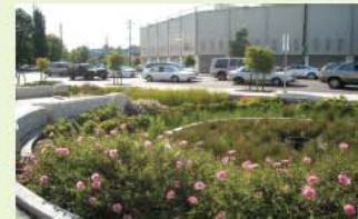
▲ This green street rain garden project was funded in conjunction with a pedestrian safety and traffic calming project.
