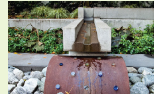
▲ A beautiful channel system directs rainwater over a lighted art installation.
