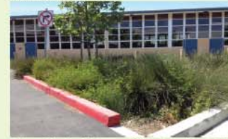
▲ Laurel Elementary School uses very little piped infrastructure in the design which helped reduce overall design and construction costs.
