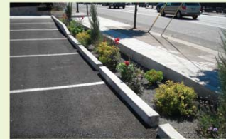
▲ A narrow stormwater planter on the edge of a parking lot.
