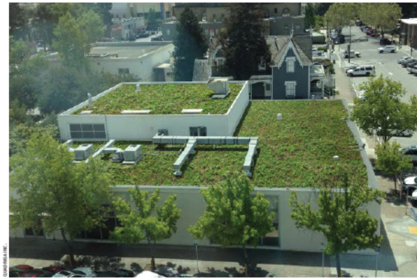
▲ RETROFIT OPPORTUNITY: The same commercial/office building rooftop with a light-weight extensive green roof application.
