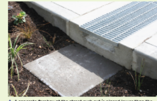
▲ A concrete forebay at the street curb cut is placed lower than the gutter grade to disperse water flow.
