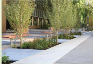
▲ This is a flow-through planter in a pedestrian plaza space that still allows for street trees.
