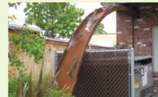
▲ A "fish ladder" conveys roof runoff into a stormwater landscape avoiding the trash receptacle area.
