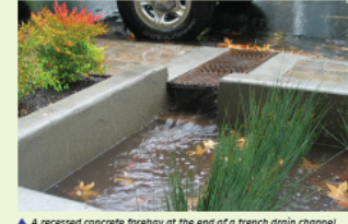
▲ A recessed concrete forebay at the end of a trench drain channel helps dissipate energy as water flows into the landscape.
