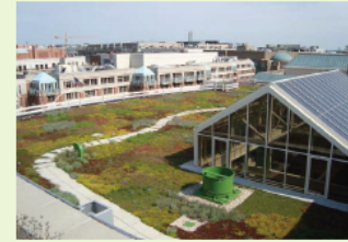
▲ EXAMPLE: An office building with an extensive green roof application.
