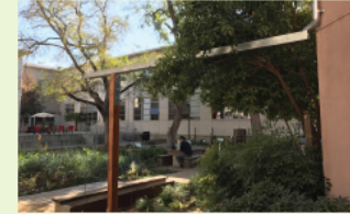
▲ A roof downspout is disconnected and routed "aqueduct style" into a rain garden at UC Davis.
