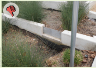
▲ Without a hard splash pad, the soil downstream of this weir is experiencing significant erosion.
