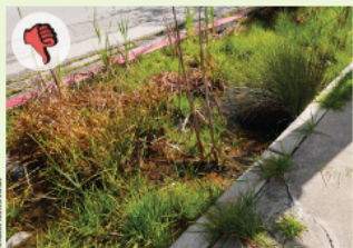
▲ Without regular weeding maintenance, a stormwater landscape can quickly be overtaken by undesirable plants.
