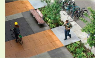
▲ Pedestrians can cross over stormwater planters using bridges or metal grates without sacrificing surface landscape space.
