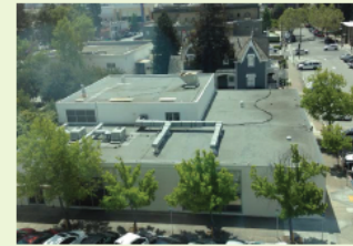
▲ EXISTING: A typical commercial/office building rooftop in San Mateo County.
