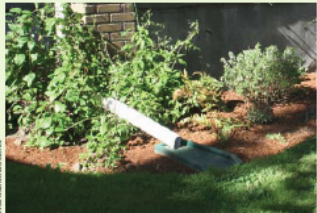
▲ A simple residential downspout disconnection directs roof runoff into a front yard.
