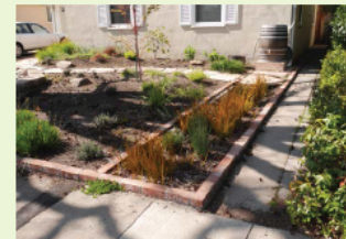
▲ EXAMPLE: An example residential stormwater planter that captures roof runoff first into a rain barrel and an excess runoff is directed to a stormwater planter.
