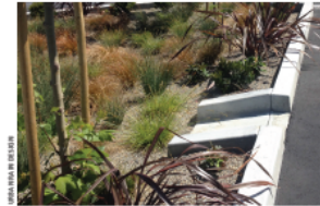
▲ This is a better curb cut option with hardscape walls and pea gravel mulch to control erosion.
