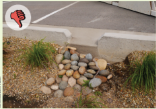
▲ It appears that the placement of rock prevents erosion, but runoff is moving around the rock and eroding soil.
