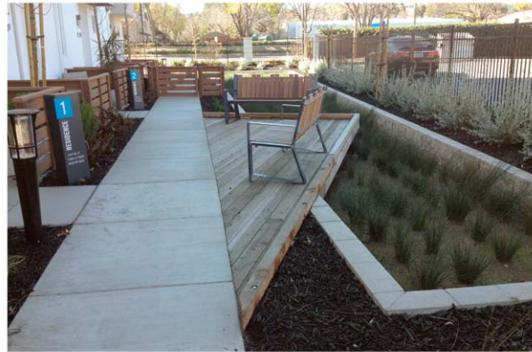
▲ This stormwater planter at a high-density residential complex accepts building runoff and integrates a seating boardwalk over the landscape.
