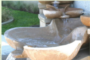
▲ An artful rainwater conveyance system from an office rooftop.
