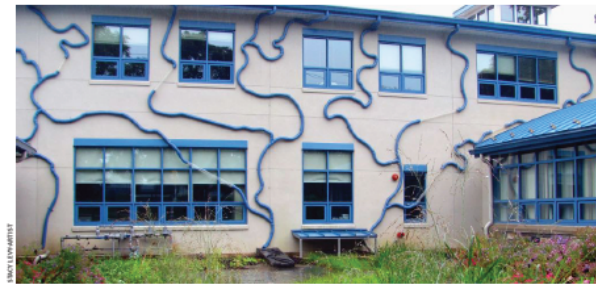
▲ An art installation that showcases the movement of water from a schoolyard rooftop into a stormwater landscape.
