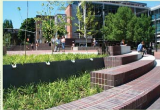
▲ A stormwater planter integrated within a series of seatwalls elegantly manages stormwater runoff in areas of grade change.
