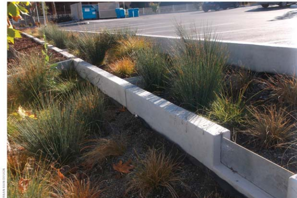
▲ This parking lot features a narrow infiltrative stormwater planter with a series of metal check dams that help slow and retain runoff.
