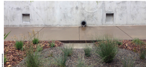
▲ This rain garden was strategically placed to capture the roof runoff from an existing roof downspout already integrated into the wall of the building.
