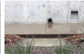
▲ A concrete splash pad and pea gravel mulch at the spill point of water reduces the potential of erosion.
