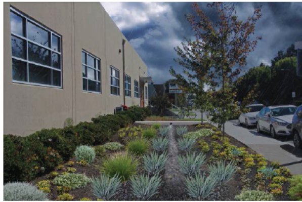
▲ RETROFIT OPPORTUNITY: The same office perimeter landscape converts un-watered grass areas into a vegetated swale with drought-tolerant landscaping. Roof downspouts direct water into the vegetated swale.
