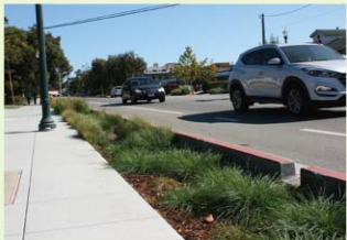
▲ This arterial street without on-street parking was retrofitted with a series of stormwater infiltration planters.
