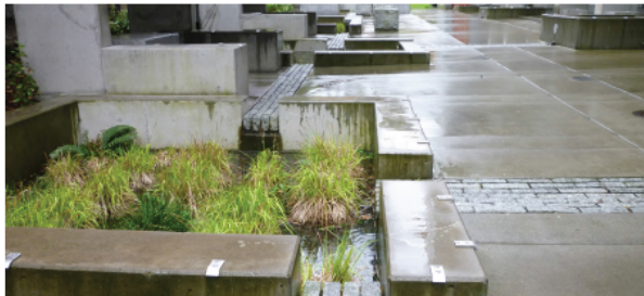
▲ This plaza space in Portland, Oregon directs roof runoff via a series of granite paver channels allowing water to flow through the joints of the pavers until it reaches the landscape.
