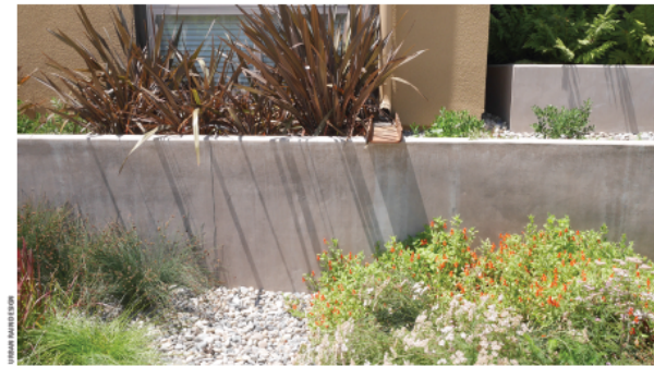
▲ A roof downspout uses a metal channel to direct roof stormwater into a planter area. It is critical that the planter maintains a rock mulch or concrete splash pad to dissipate the vertical energy of water spilling into the landscape area.
