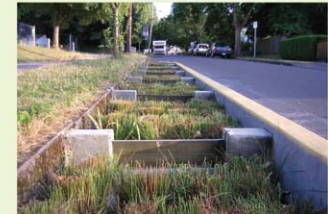
▲ EXAMPLE: This neighborhood connector incorporates a vegetated swale with check dams to reduce velocities on a sloping street.
