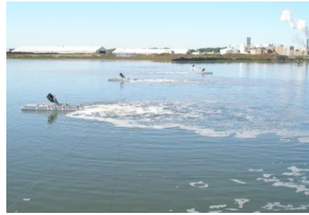
Industrial Wastewater Treatment
