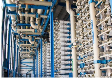
Industrial Water Treatment
