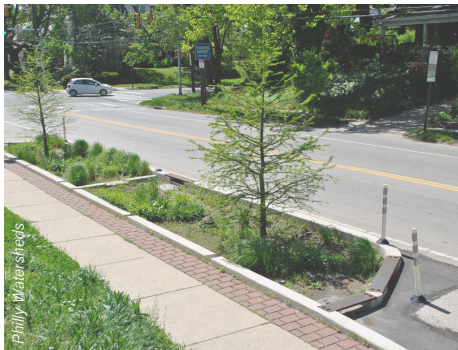
Bioretention planter bump-out, Philadelphia PA
