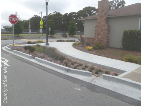
Safe routes to school stormwater curb extension, San Mateo CA
