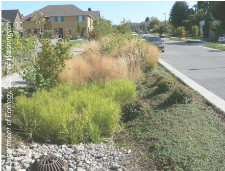
Bioretention planter, Washington
