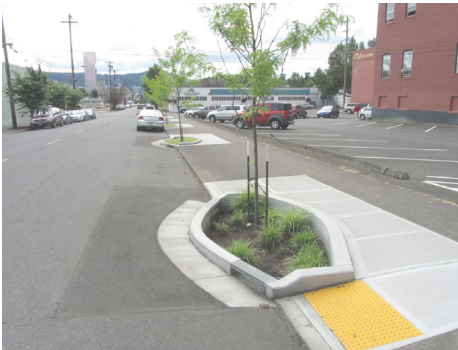
Stormwater Tree Well
