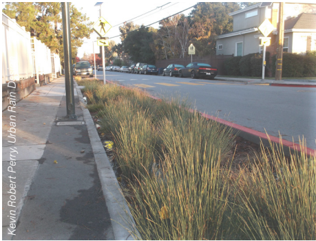
Bioretention planter extension
