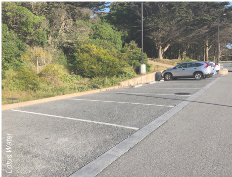
Permeable pavement parking spots, Beach Chalet, San Francisco
