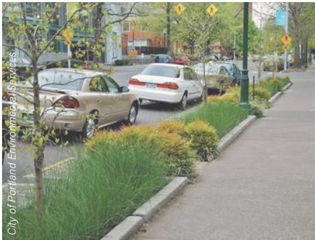
Bioretention planter buffer, Portland
