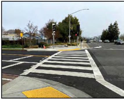
HIGH-VISIBILITY CROSSWALK/CURB RAMPS
