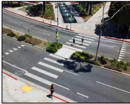
MEDIAN CROSSING ISLAND
