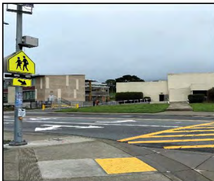
RECTANGULAR RAPID FLASHING BEACON (RRFB)
