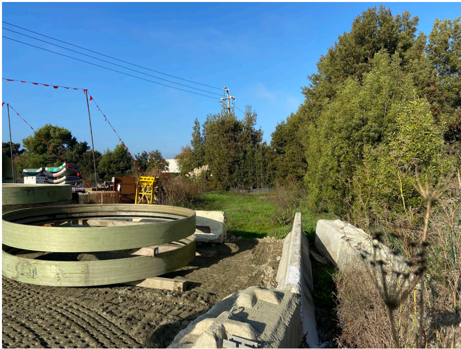
Figure 3-12. Staging area near channel. Overhead utilities are observed.
