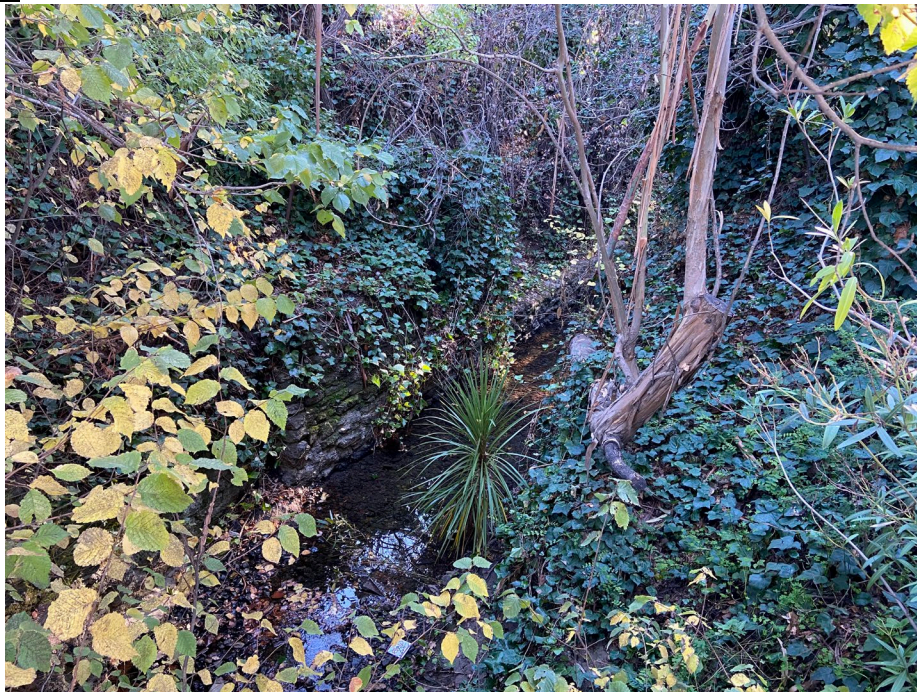
Figure 3-29. Channel upstream of headwall to culvert.
