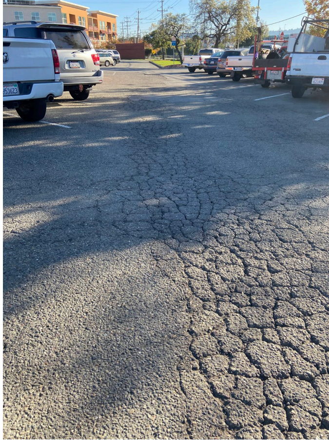
Figure 3-26. Pavement condition of parking lot and drainage pathway.
