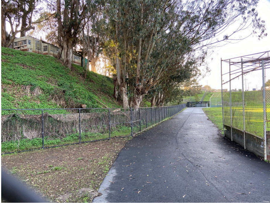
Figure 3-42. Access driveway and the existing pump station.
