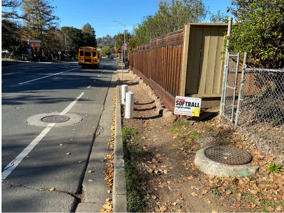
Figure 3-20. Diversion location and pipe confluence (looking north).
