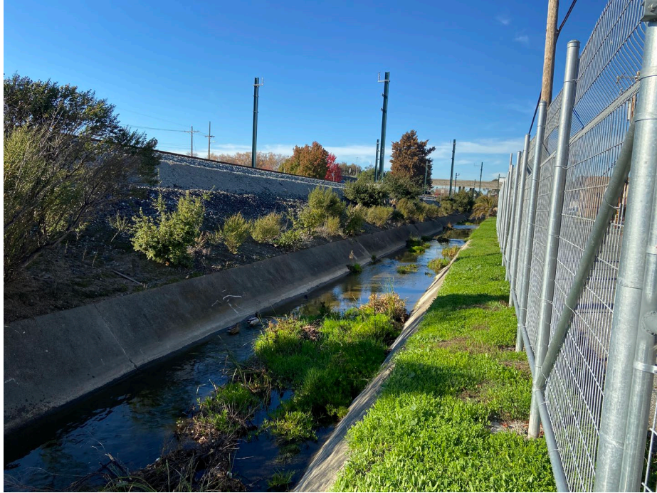
Figure 3-24. Trapezoidal channel to be diverted to storage.
