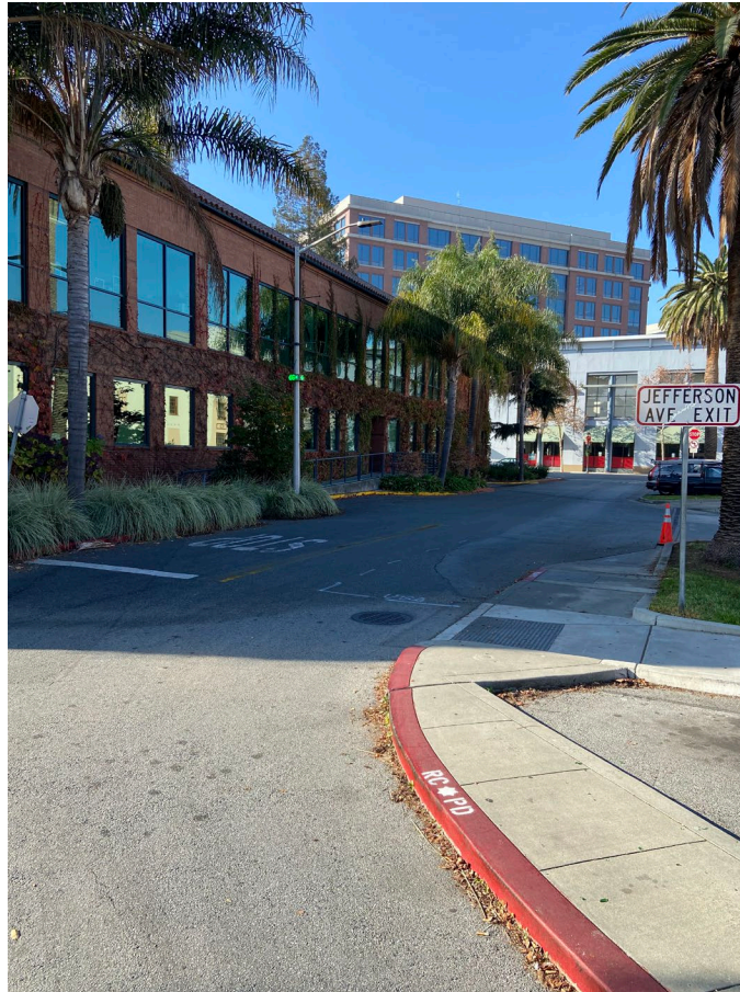
Figure 3-14. Existing site access and storm drain merge location. Diversion within this vicinity.
