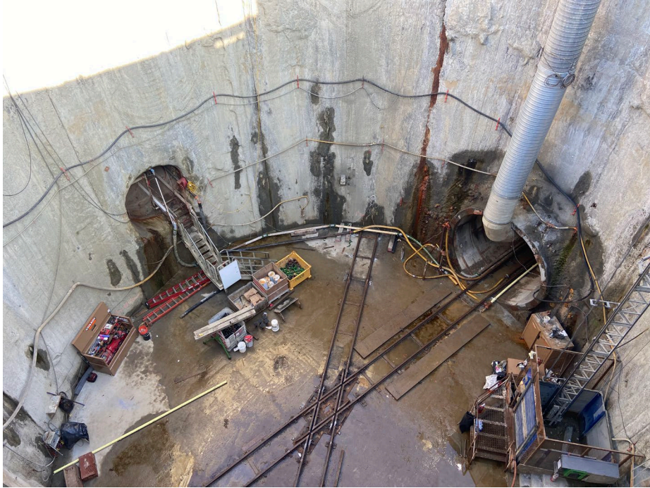
Figure 3-11. Present construction activities for sewer line.
