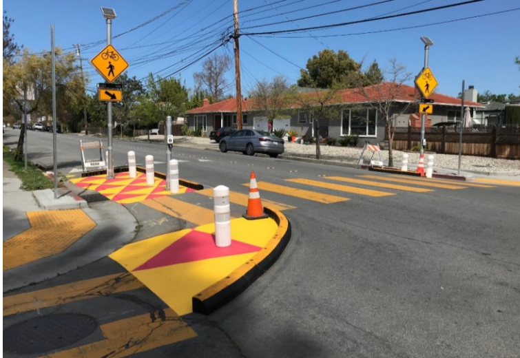
Figure 3: Installation of RRFB and quick-build curb extensions at Vera Ave/Hudson St Intersection.
