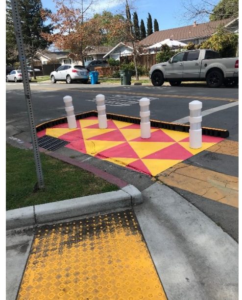
Figure 4: Curb extensions are installed at three major intersections on the Vera Avenue.
