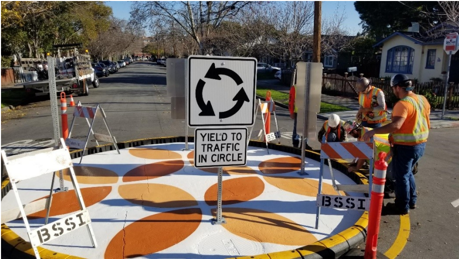
Figures 1 & 2: Five traffic circles are installed along the Vera Avenue with quick-build materials. The traffic circle patterns are submitted by the neighborhood residents and implemented by the construction contractor.
