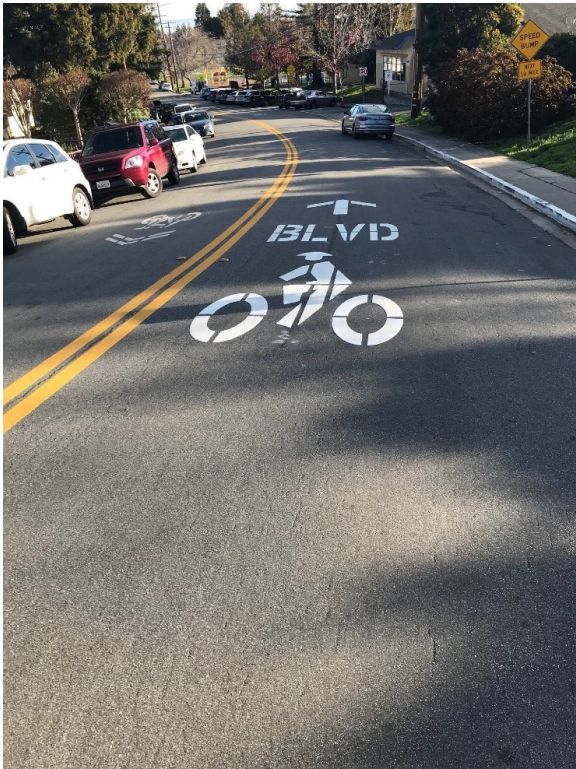
Figure 5: "Bike Boulevard" pavement markings along the Vera Avenue.
