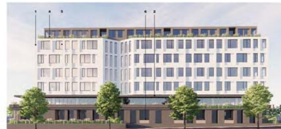
RESIDENTIAL VIEW FROM SPRUCE AVE
