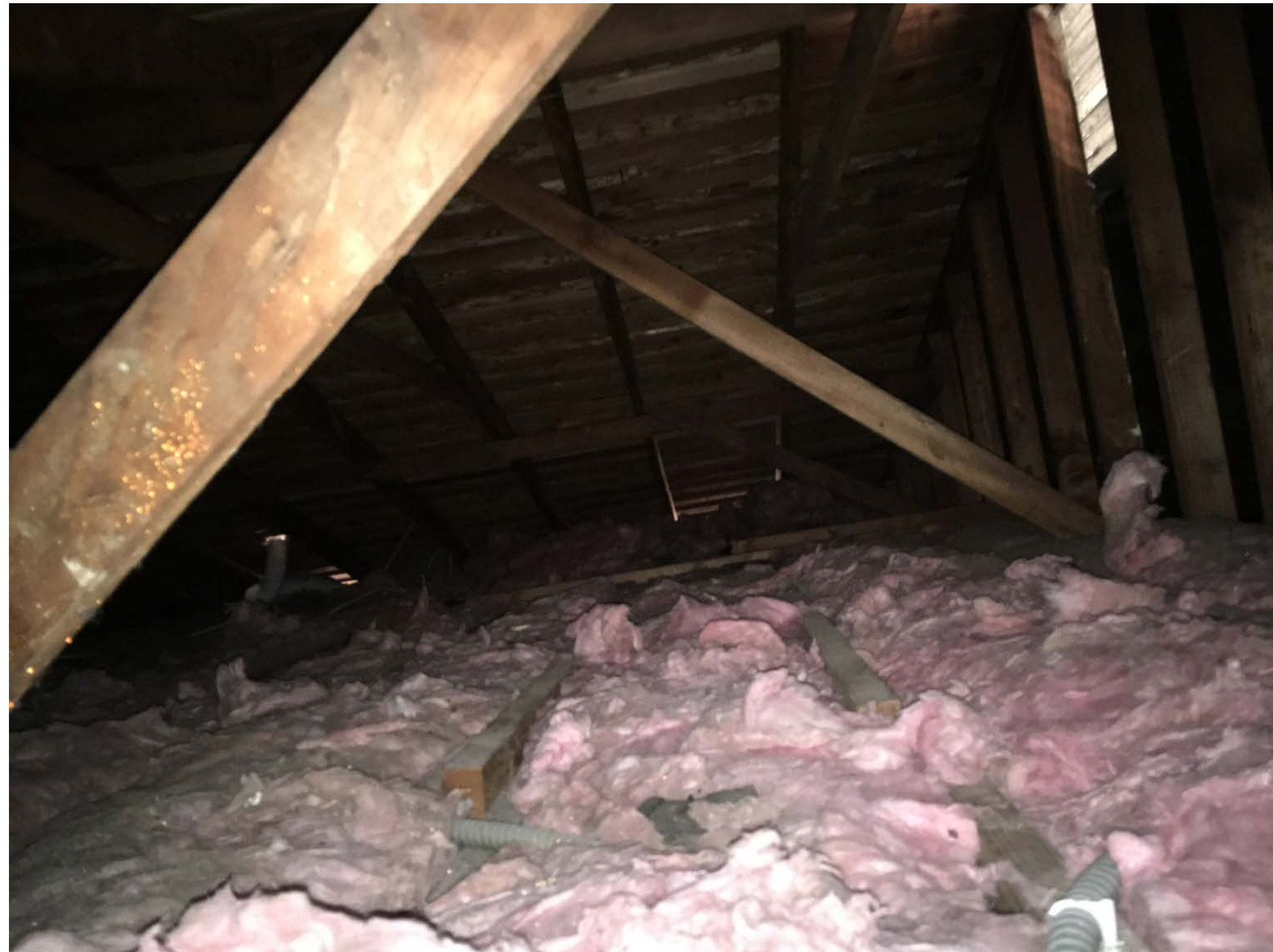
Today: Attic, R-19 insulation Recommend: R-38
