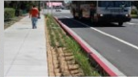
12 San Mateo, Delaware St Green Street
