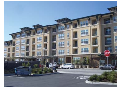
Over 700 units have already been built at the former U.S. Navy West Div site, and construction of 350 additional housing units is underway.
