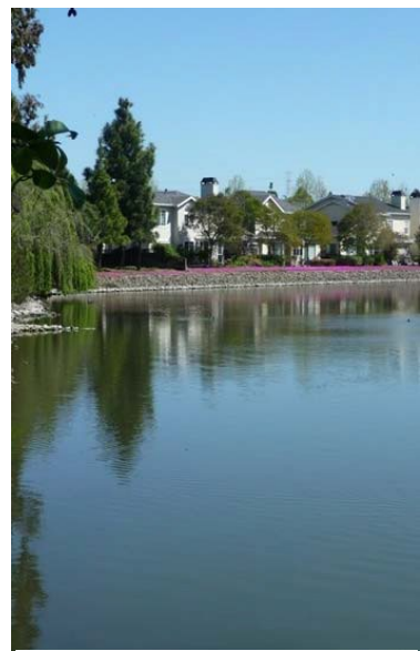
The lagoons in Redwood Shores function as stormwater detention basins.
