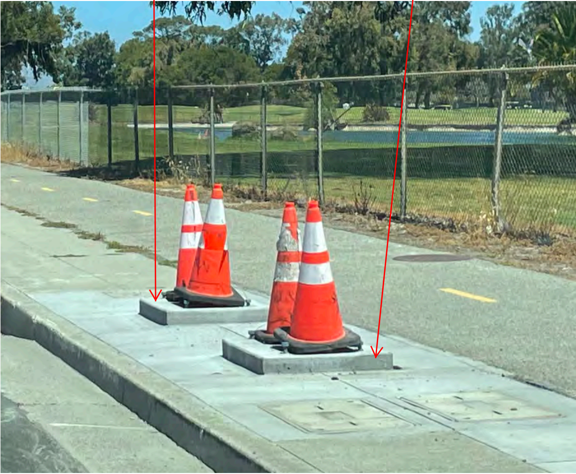
TOLLING ITEM #16: FOUNDATION PAD FOR MODEL 332L CABINET FOR ELECTRONIC TOLL SYSTEM
