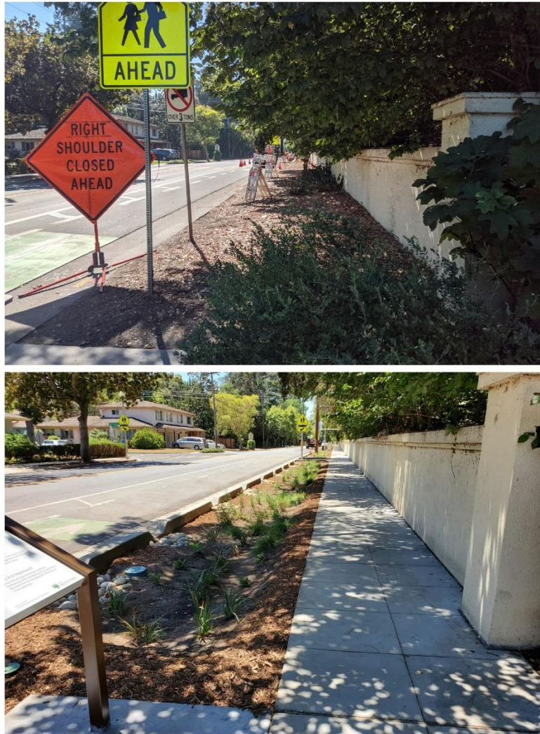
Figure 11. This street transformation in Menlo Park, San Mateo County, demonstrates how planned infrastructure projects such as adding a sidewalk, repaving, or replacing pipe represent opportunities to add green infrastructure/flood mitigation. The OneWatershed framework can identify such opportunities for layering benefits and reducing agency/community shared-risk.
