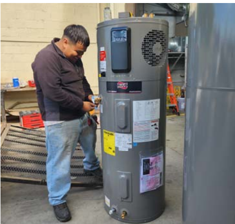
A new heat pump water heater being installed at the County corp. yard.
