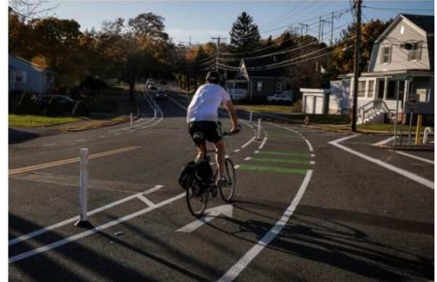
Example of a Feasibility Study – Using Temporary Paint and Plastic Delineator Posts To Alter Roadway Cross Section
