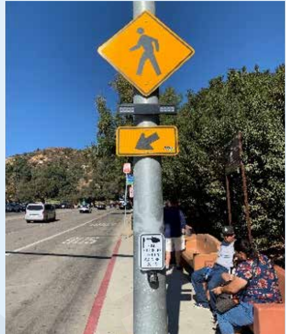
Rectangular Rapid Flashing Beacons (RRFBs)
