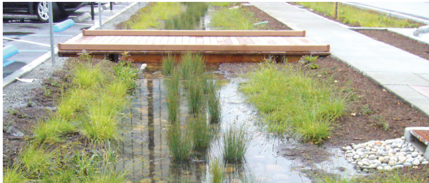
Bioretention/rain garden (Image credit: C/CAG)
