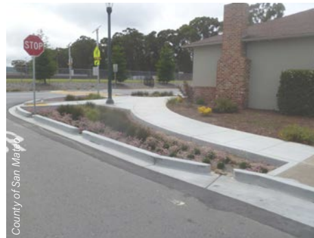
Safe routes to school stormwater curb extension, San Mateo CA
