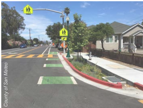
Safe routes to school stormwater curb extension, Burlingame CA
