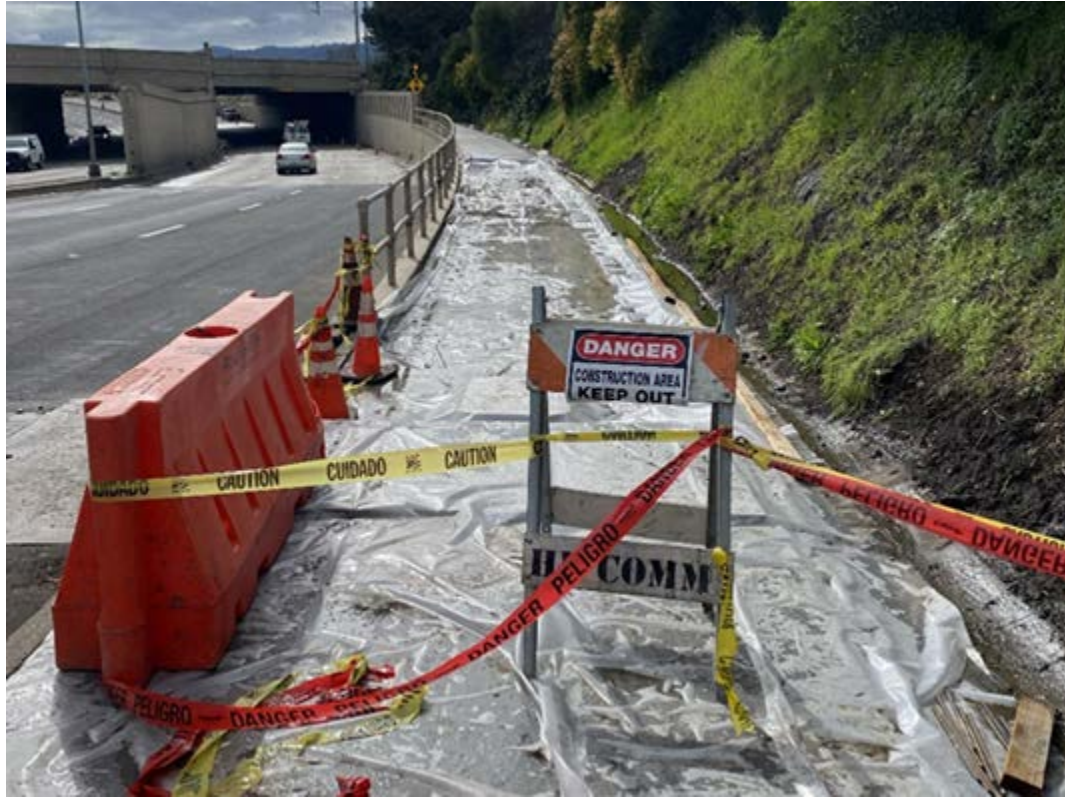
Utility Trench Excavation installation along walkway (Airport Blvd)
